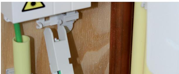
The AU-FTU forms the link between the passive optic fiber network and the operator's active part. The end-user can easily set up the connection between the passive optic fiber network and the active equipment, such as a fiber optic modem, CPE or NT, using a standard patch cable provided with the supplied insertable modules, without any possibility of error or fault.
